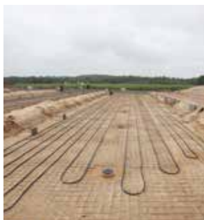
Slurry cooling systems under construction
