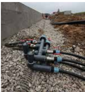
Slurry cooling systems under construction
